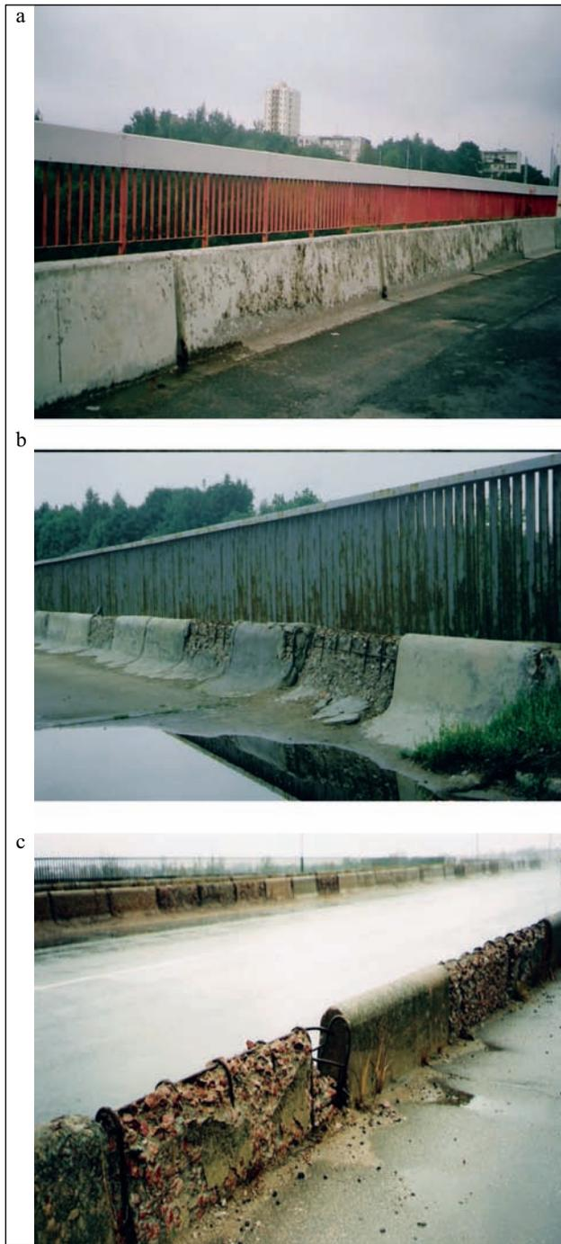
Fig 5. Typical deterioration of RC safety barriers after 8 (a), 26 (b), and 36 (c) years in service
