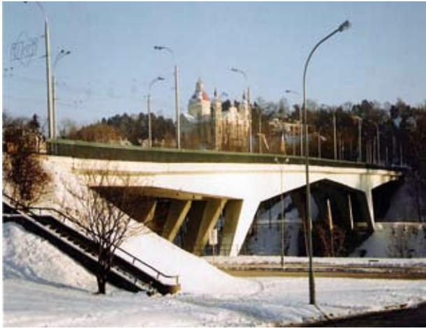
Fig. 1. One of the first PC precast segmental bridge with concrete joints over Neris River (bridged in 1965)
