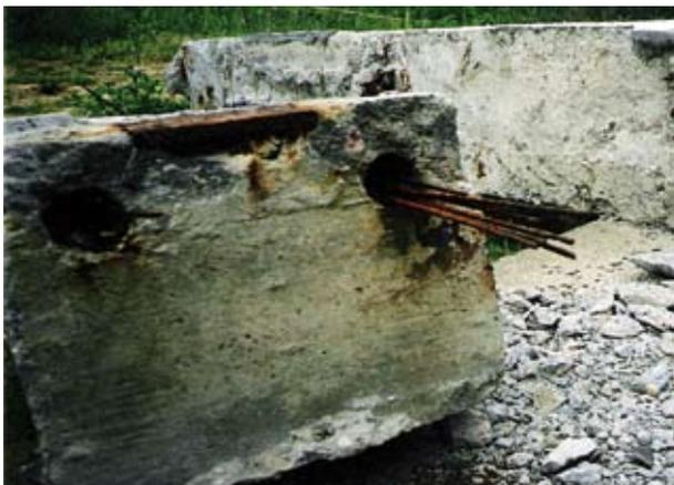
**Fig. 6.** Failure of bridge staircases due to corrosion of prestressed tendons in the dry joints
