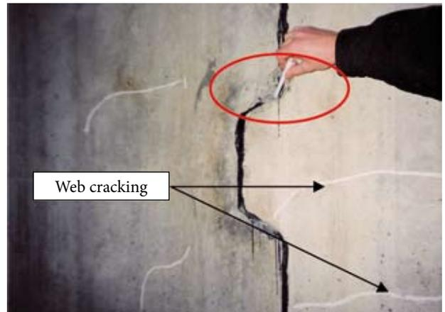
**Fig. 8.** Spalling of the concrete at the joint and concrete cracks in the box girder web
