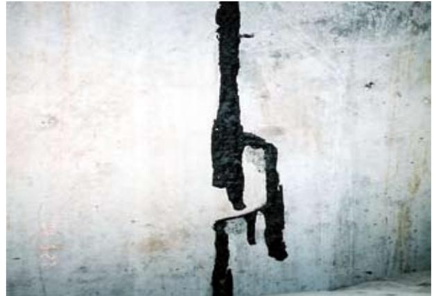
**Fig. 7.** Flowing out of the epoxy glue from the too large joint
