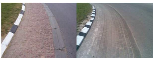
Fig. 13. The damaged road kerbs by riding up on the block-paved circle, the broken inner road kerbs at joints
