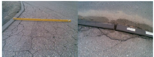
Fig. 10. Road structures damaged due to their unconformity to traffic and operational conditions
