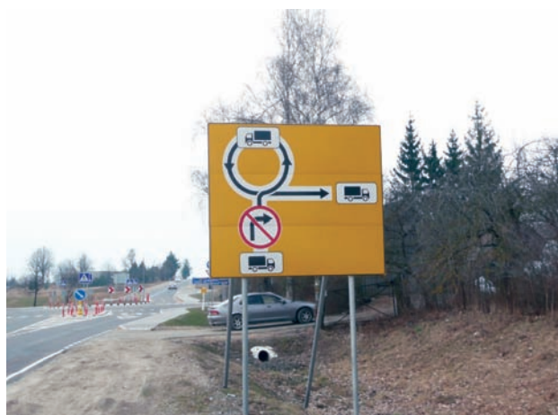
Fig. 7. The roundabout where the heavyweight vehicles are not able to make the right turn
